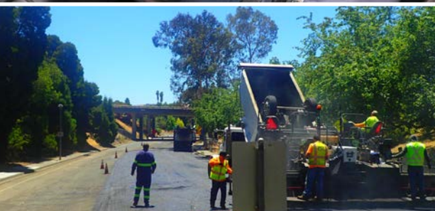
Southampton Road Replacement
